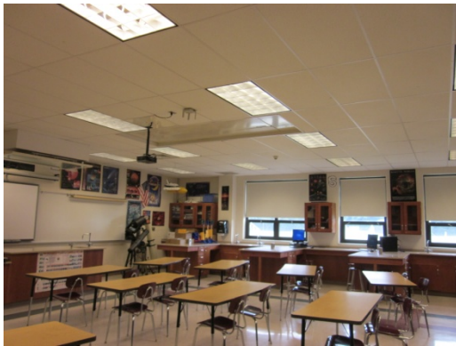
Chatham HS- Classroom with Manual Light Switch
