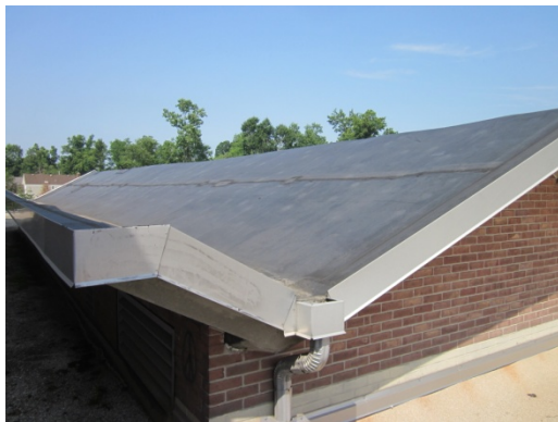
Chatham High School Cafeteria Roof
