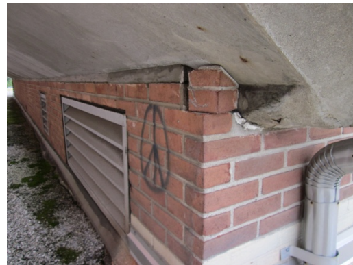
Chatham High School Roof
