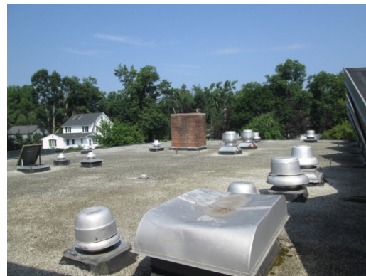
Chatham High School Kitchen Roof
